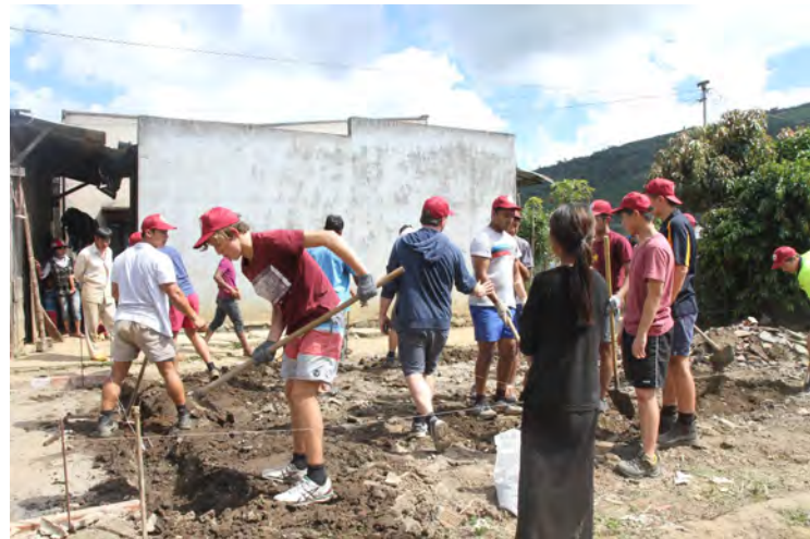
Above: Digging and preparation for the laying of house foundations
