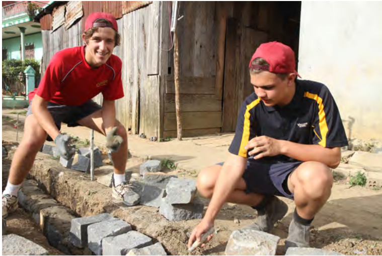
Above: Laying house foundations
