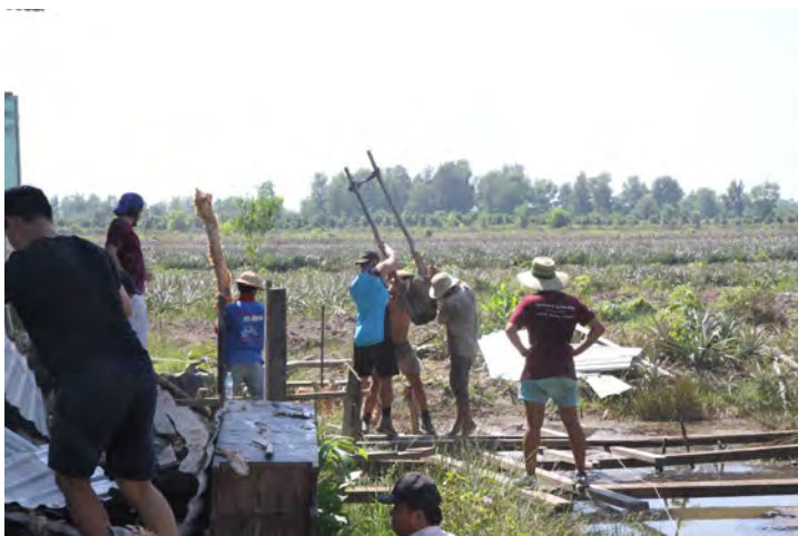
Above: volunteers lay house foundations
