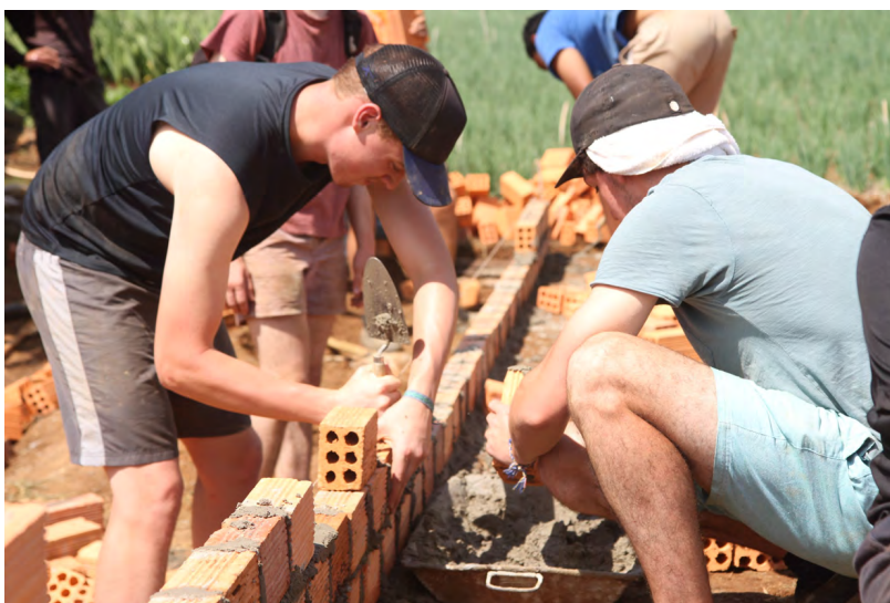
Above: brick laying for a house in K'long
