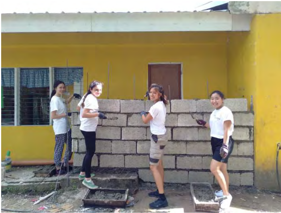
Above: building toilets for children at Vilialimpia Elementary School
