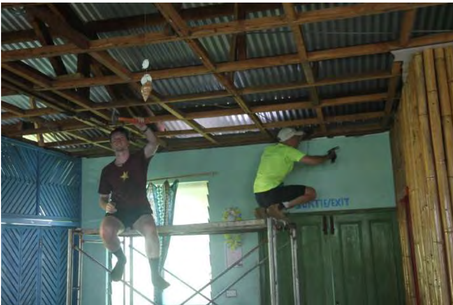
Left: refurbishing the school
