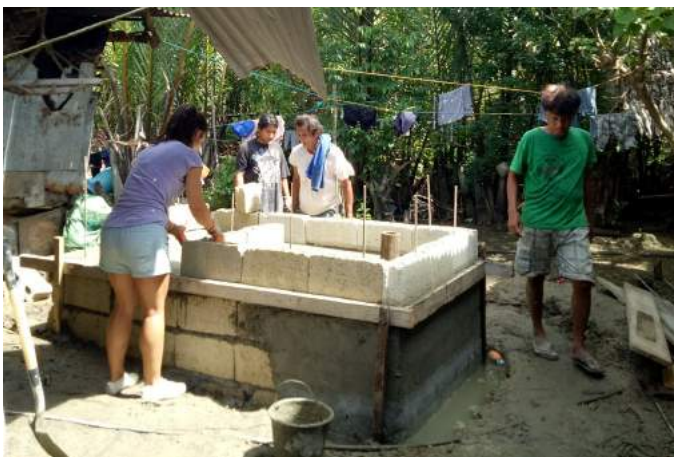
Left: volunteers constructing toilets
