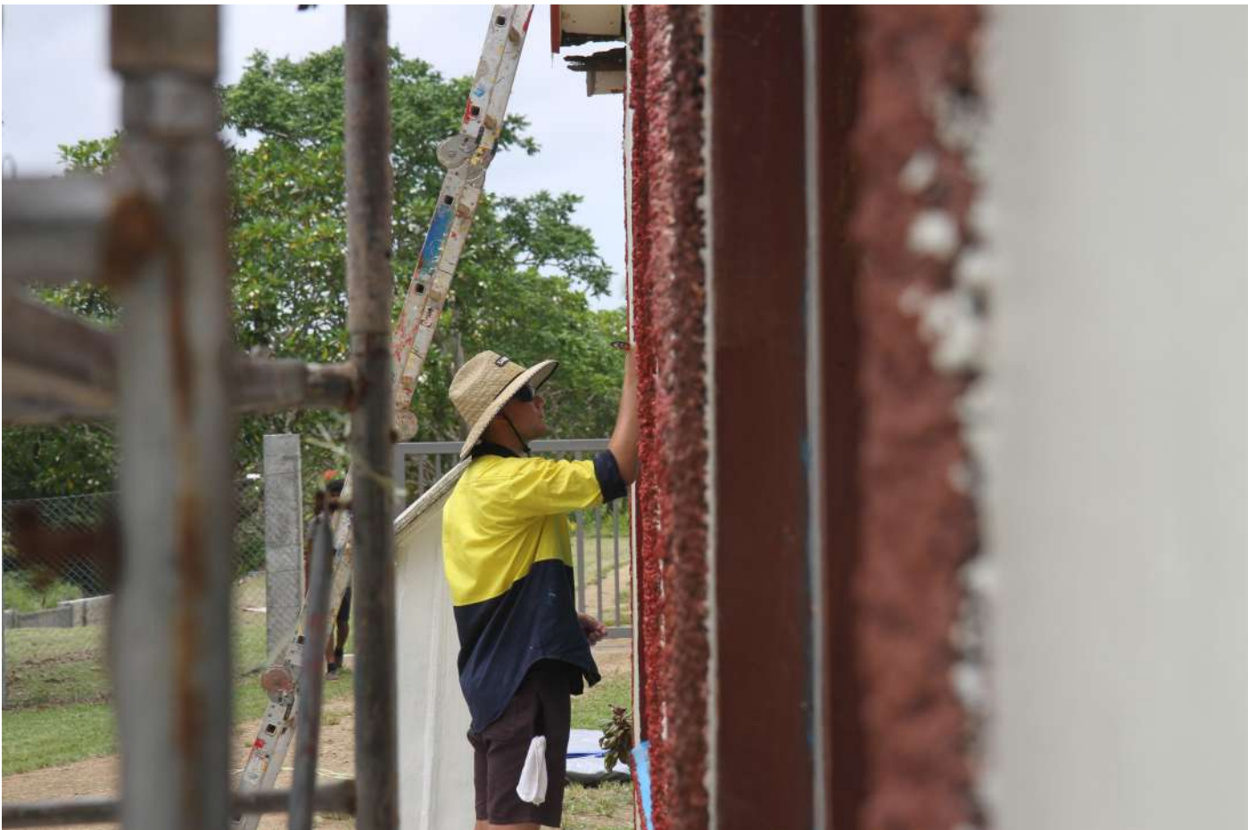
Below: repainting the San Michel church
