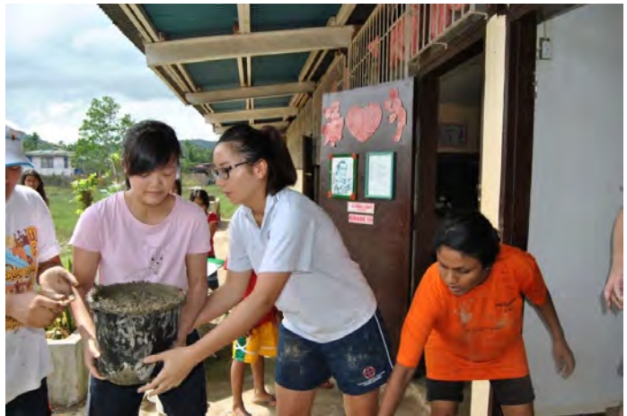
Below: volunteers repair a damaged school building.
