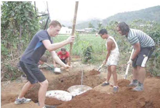
Above: volunteers install septic tanks for newly built toilet blocks
